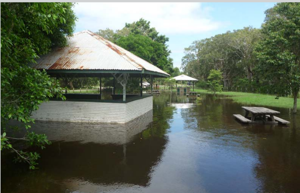
Photo: 2013 - Flooding at Mungo Brush
