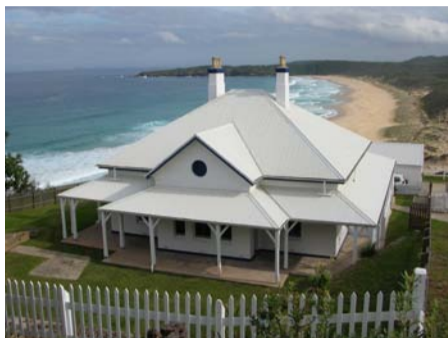
Renovated Head Keepers cottage at Sugarloaf Point Lighthouse, Seal Rocks
